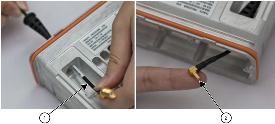
Figure 93: GNSS Cable Installation
